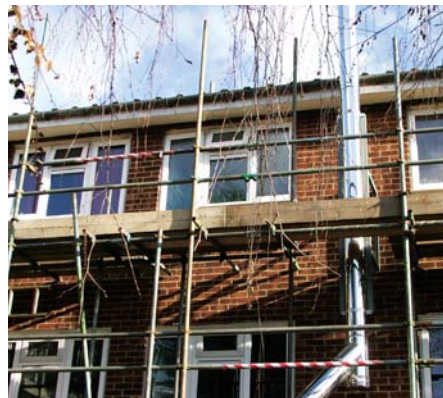
New flues are being installed at Sanford.
