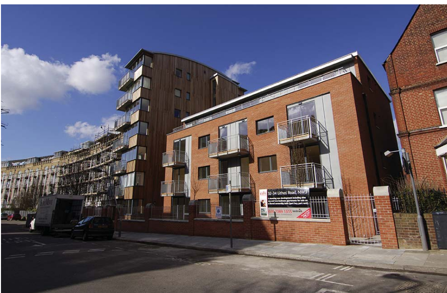
CRISH's new block in Camden is built in brick, while the tower block has red cedar timber cladding.
