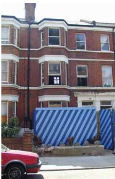
The work involves refurbishment and rebuilding
