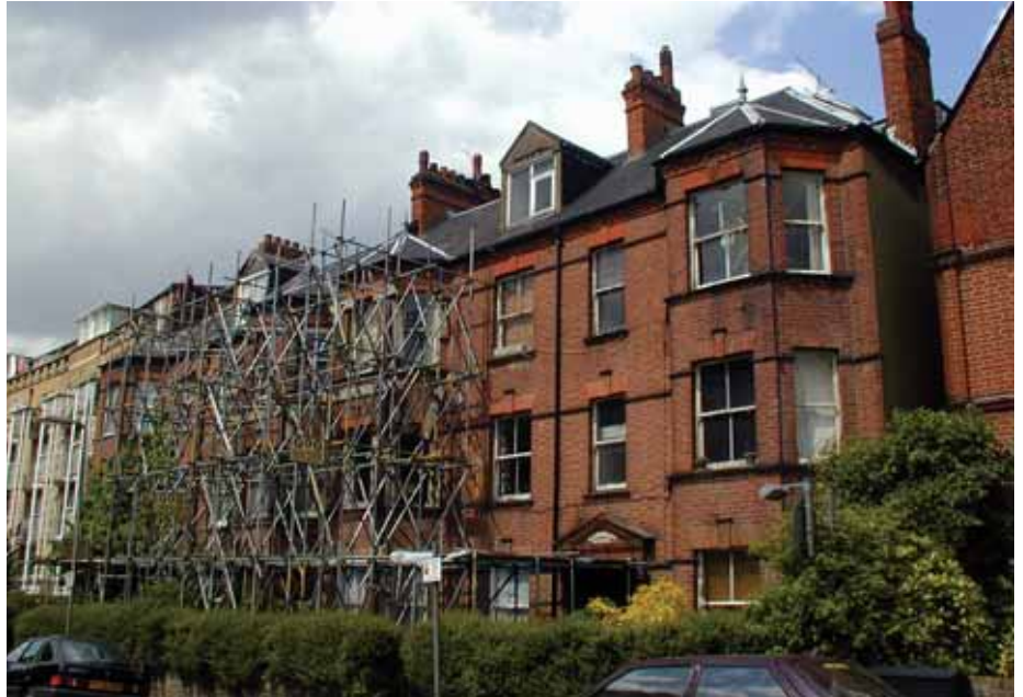
Demolition is now complete and the project is on track
